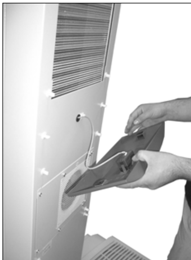
Fig. 64: Take off the infill panel
